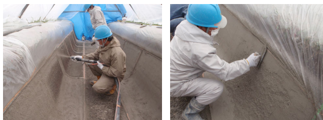
Fig.1 表面被覆工の着手前と完了後の事例 Cases of pre-construction and post-construction
