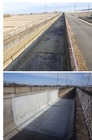
Fig.1 表面被覆工の着手前と完了後の事例 Cases of pre-construction and post-construction
